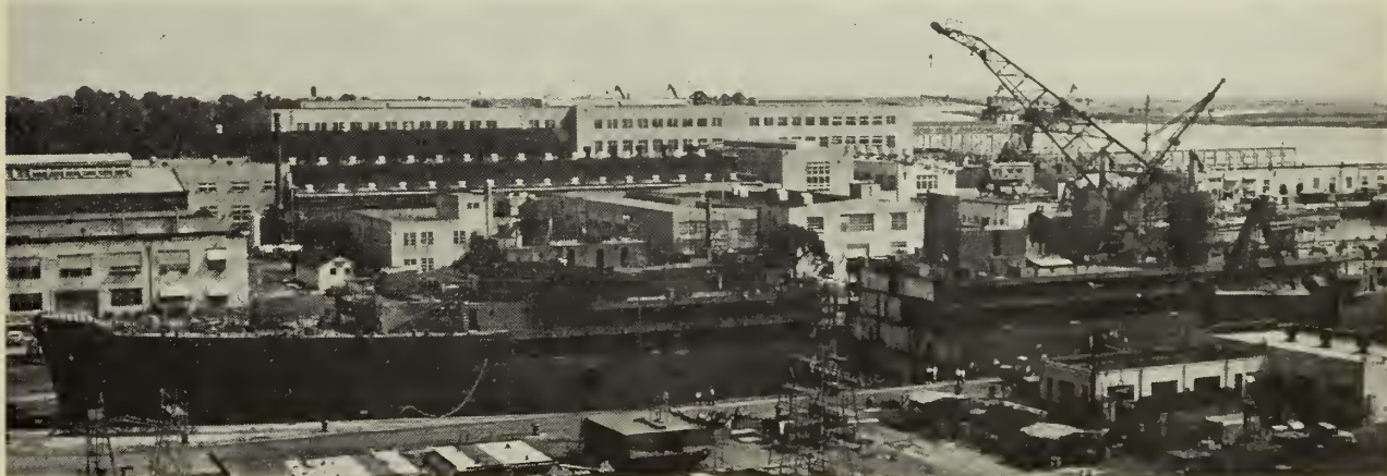
MID-RIFF — USS Proteus (AS 19) lies in drydock at Charleston, split in half to add new midsection that will equip her with special shops and gear to serve as a Fleet tender to the Navy's first squadron of nuclear submarines.
